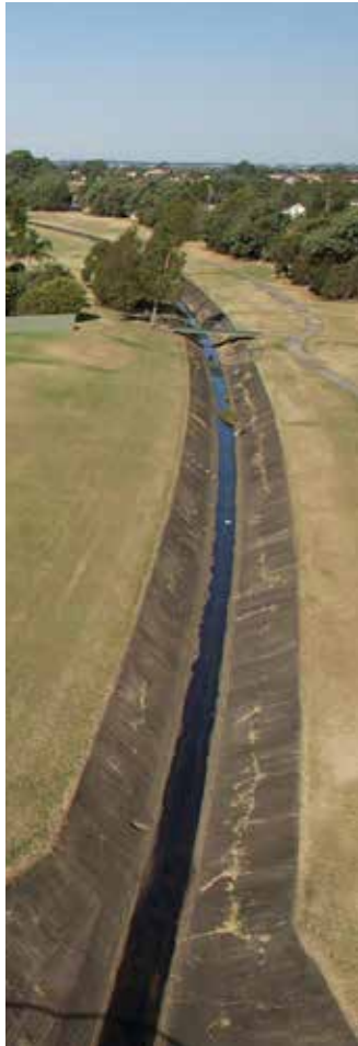
The existing concrete stormwater channel.
