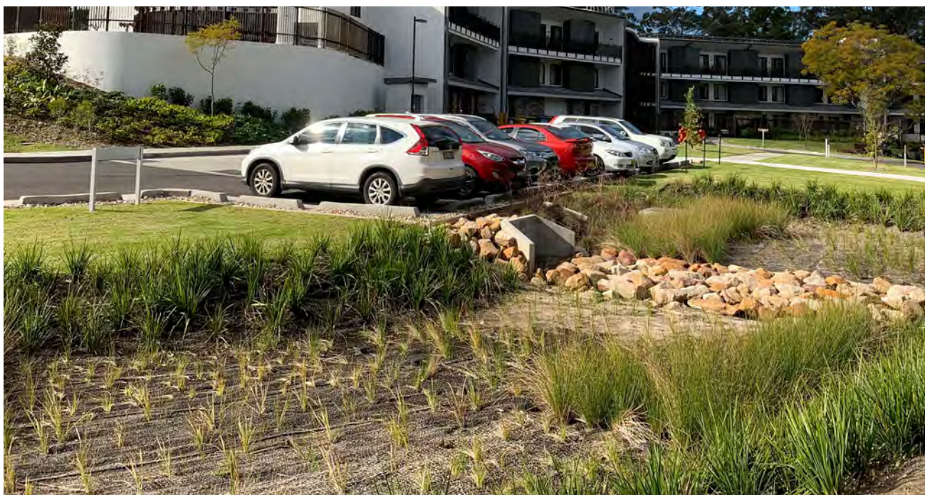
Fig 12.9.A Sensitive landscaped stormwater detention in the gardens of a residential care facility
