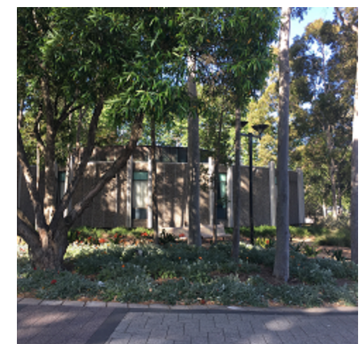
7. Heritage structures (council owned)
