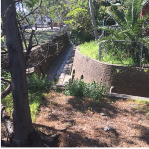
7. Salt Pan Creek stormwater channel
