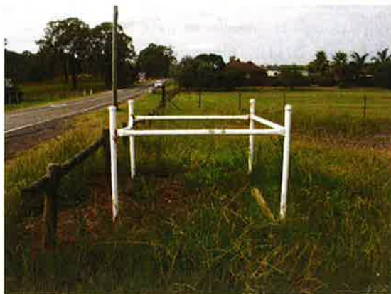
Figure 5.73 Post-and-rail fence; view from the north.
