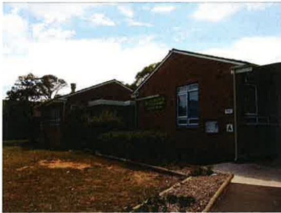
Figure 5.117 Building A, Administration.
