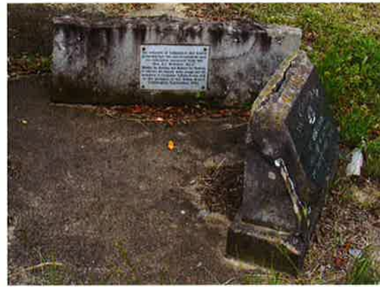
Figure 5.80 The sandstone base of the memorial is suffering significant deterioration, including contour scaling.
