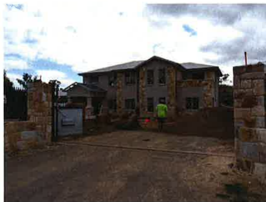
Figure 5.202 Child care centre under construction.
