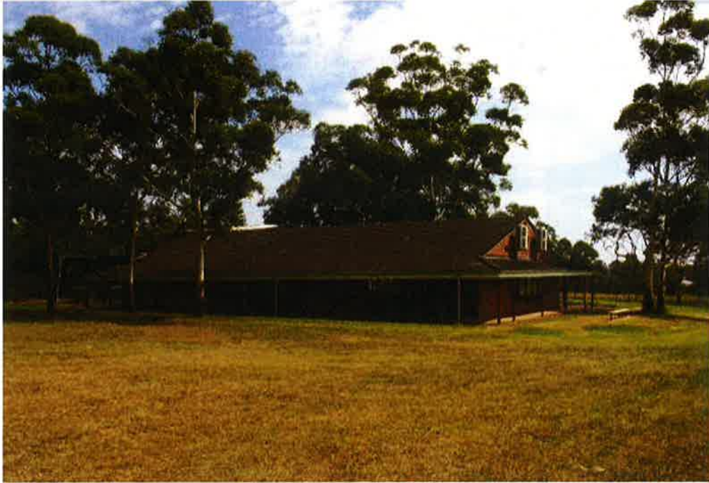
Figure 5.119 Building E, Library.
