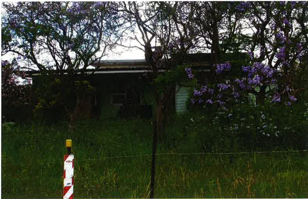
Figure 5.84 Front of dwelling, 1720 Camden Valley Way.
