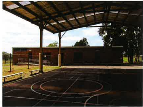
Figure 5.118 Building C and sports court.
