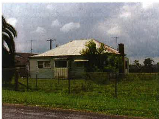
Figure 4.24 Weatherboard house at 45 Gurner Avenue.
