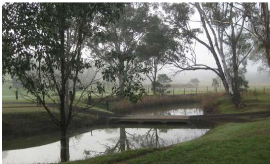
Figure 19. Section of Killarney Chain of Ponds with recently constructed causeway.
