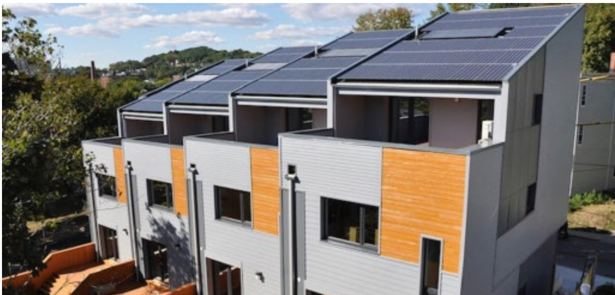
Figure 3-124 Roof mounted photovoltaics should be integrated into the design of the dwelling
