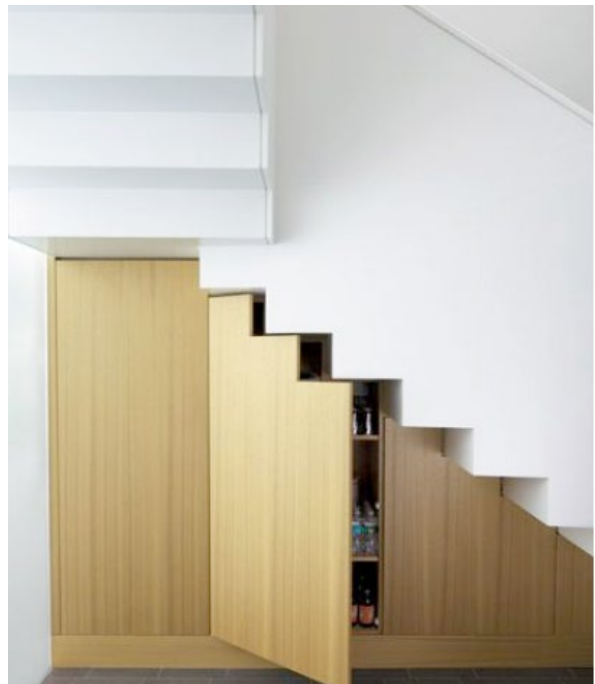
Figure 3-85 Storage space under stairs
