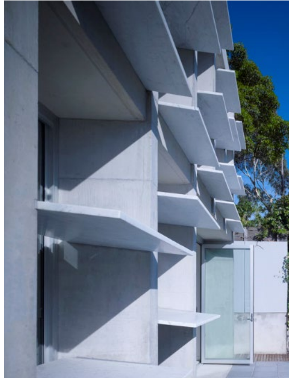
Figure 3-125 Light shelves can reflect sunlight deeper into rooms and provide shade from summer sun
