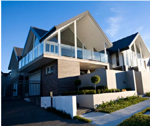
Figure 3-108 Roof form expressed
