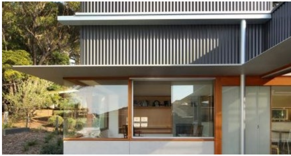
Figure 3-115 Awnings provide shelter and add articulation
